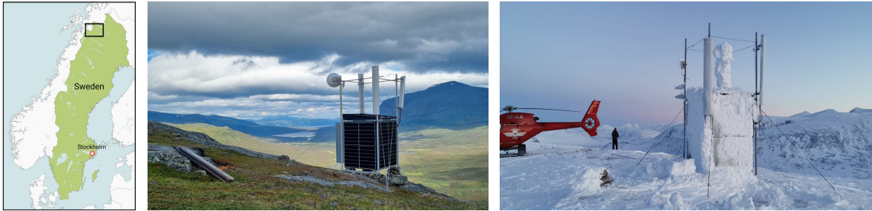
Fig. 4. Network of autonomous cellular BSs (no roads, no wired (fiber) backhaul, and no electricity grid) connect today the indigenous Sami people in their summer villages in the valleys of Arctic Sweden. Left: map with an indication of the region. Middle: summer impression (photograph: Jon Anders Svonni). Right: winter impression (photograph: Håkan Enoksson).
